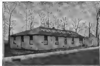
INDIANAPOLIS PLANT NO. 2
